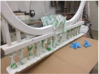
were replaced; the ornamental columns were stripped and repaired and then a paint underlayment added to increase longevity before applying the exterior paint; the floor sills and joists were replaced with pressure treated wood.
