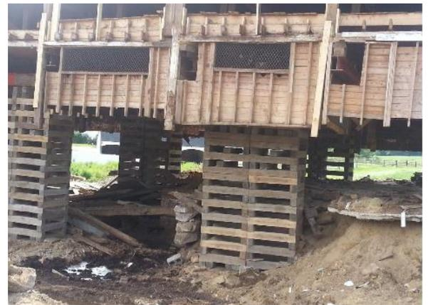
The rotting away of the undercarriage of the barn, caused by years of wet animal manure being dropped below, where there was already a problem with lack of drainage, made it necessary to remove the basement and place the barn at grade level.
