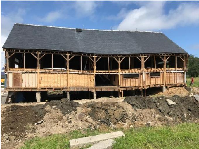
The underpinnings were replaced and the building is now back on the ground on a new foundation. The side boards are being put on as they work to button it up before the gales of winter come
